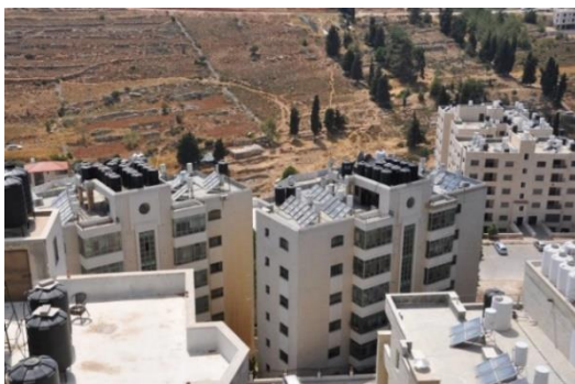
Private tanks are increasingly deployed on roofs of Ramallah buildings to provide much-needed water. Credit: Mohammed Najib/Al Jazeera.
